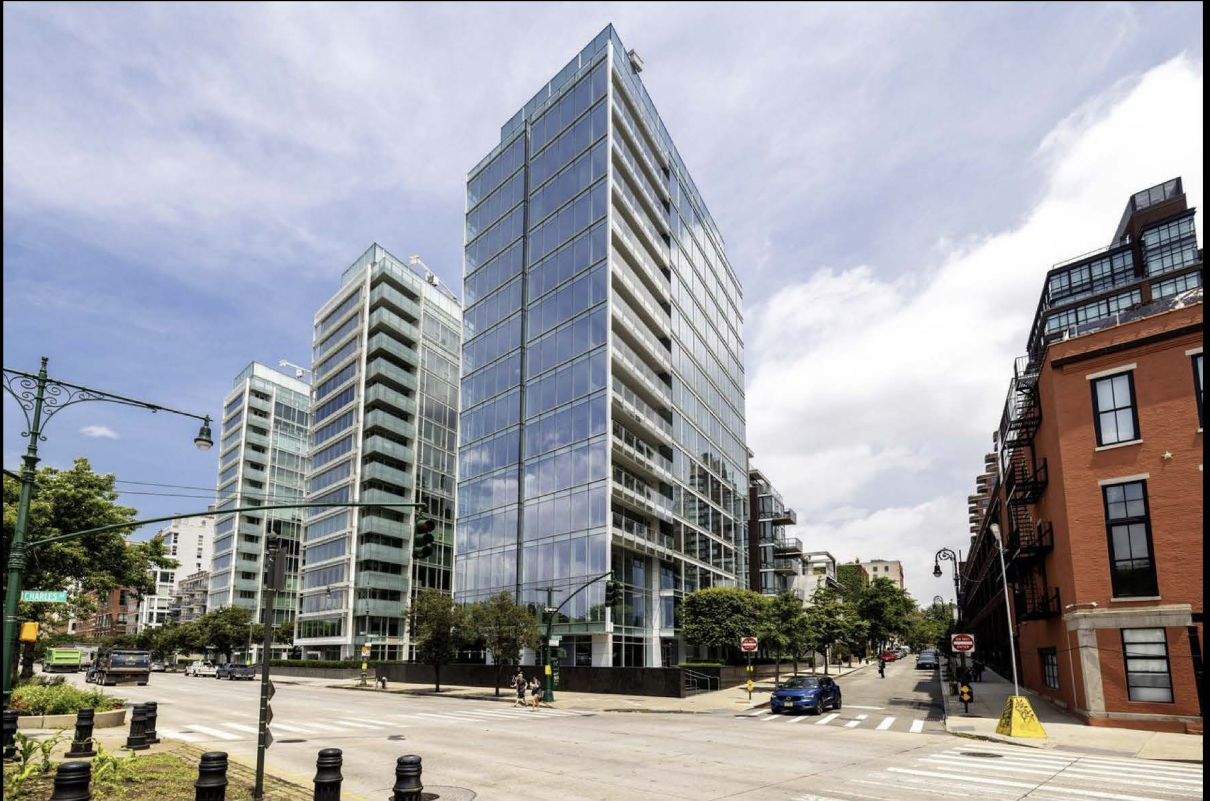
Three Richard Meier-designed buildings line the West Side Highway; on the right is 165 Charles. Credit: DOROTHY HONG FOR THE WALL STREET JOURNAL
